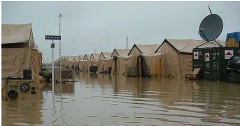
Flooding at K2 Tent Camp. The entire camp was covered with stones and gravel to 'cap' the contaminated ground. However, when rain or flooding occurred the contaminants would rise to the surface and spread. (photo provided by CSM Ret Jose Silva)
